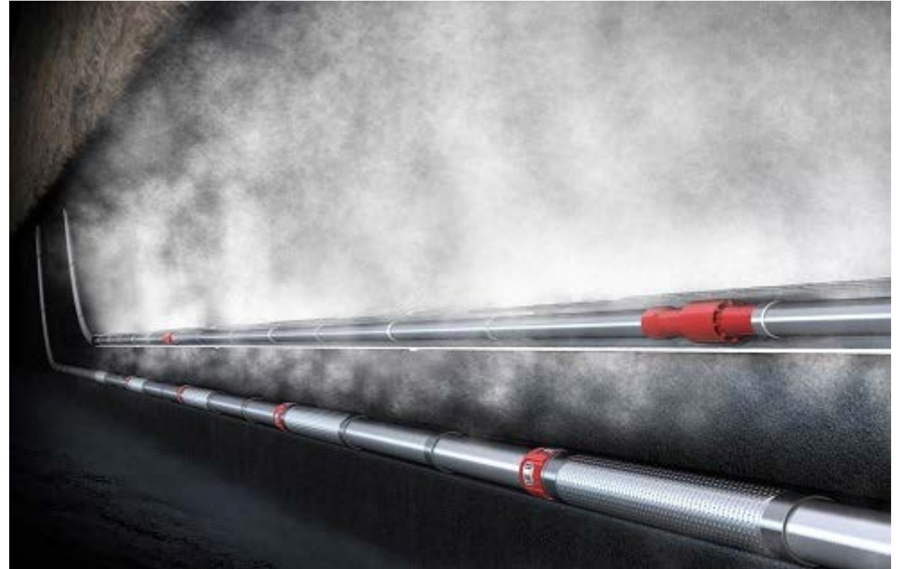
FCDs Deployed in a SAGD Well (Halliburton)
